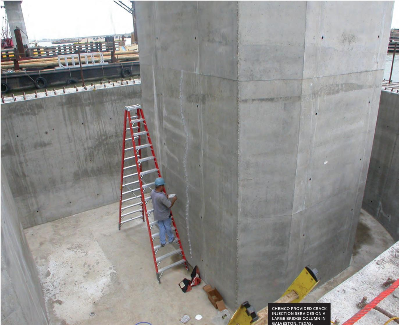
CHEMCO PROVIDED CRACK INJECTION SERVICES ON A LARGE BRIDGE COLUMN IN GALVESTON, TEXAS.
