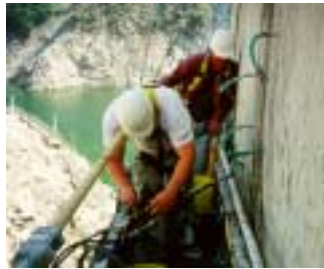
Pacoima Dam injection
